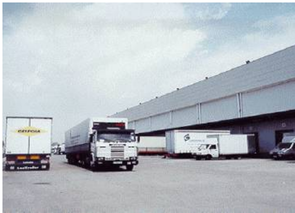
Warehouses with raised docking bays
