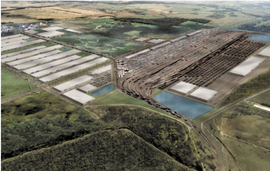
CenterPoint Intermodal Center – Elwood, Ill.
