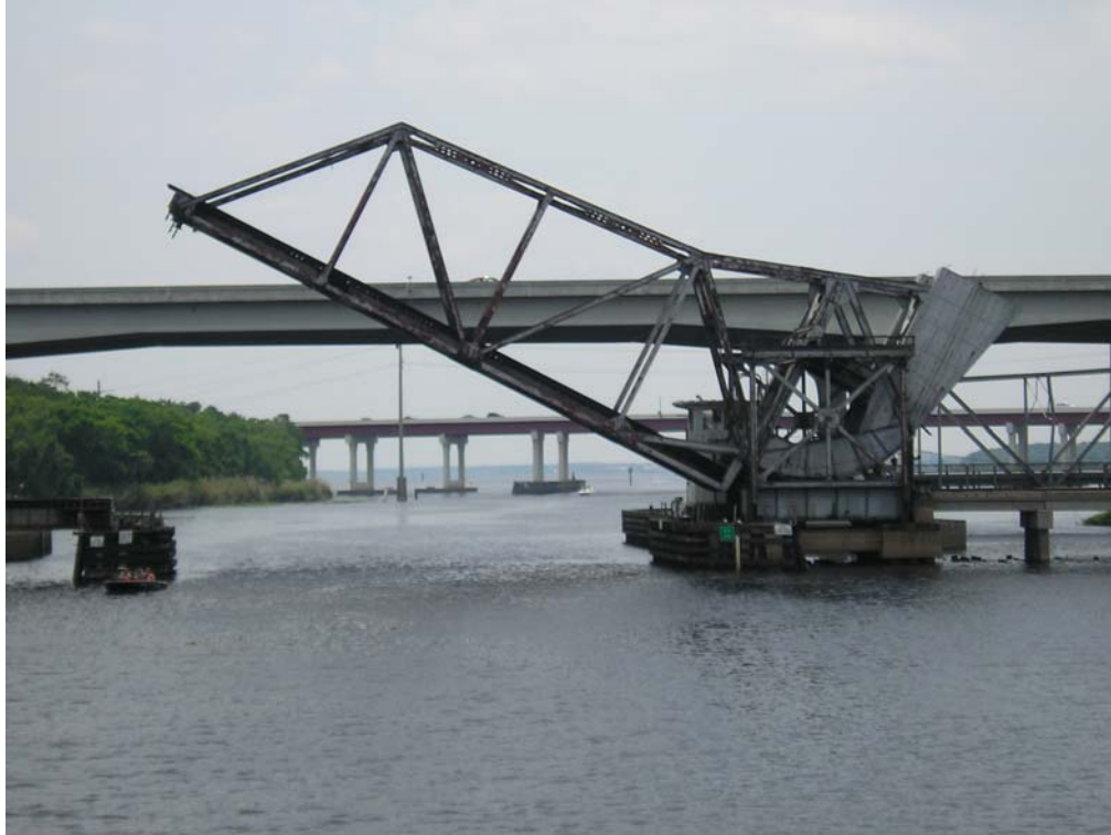
Figure 4-11 Existing CSXT Lift Bridge at St. Johns River
