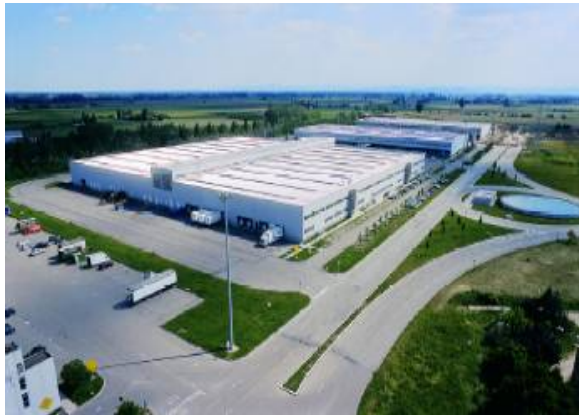
Large-size warehouses for logistical activities
